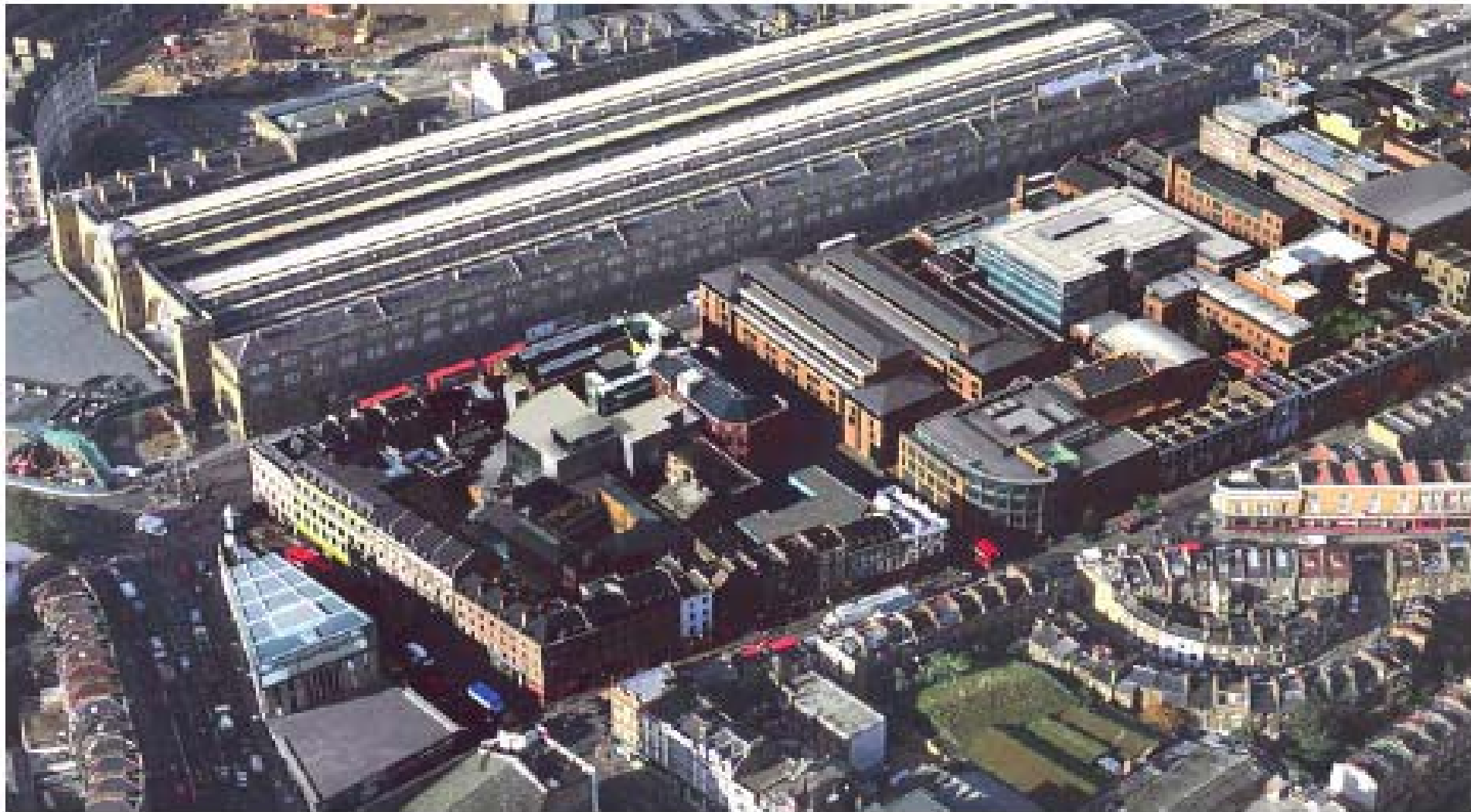
Figure 22, Regent Quarter future view of the site (source data: Brochure one master planning, P&O – RHWL Architects, August 2001)
